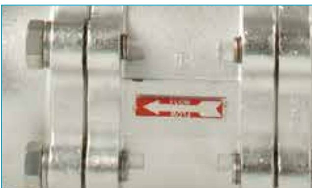
Indicator on valve body
